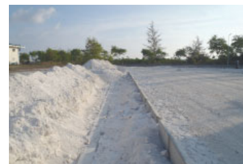
Hulhumale Road Development Project
